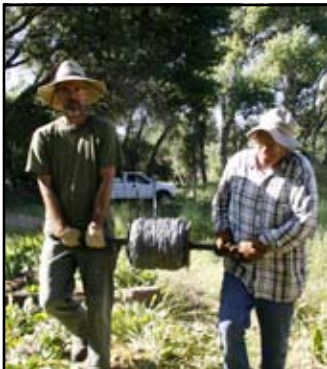
Sean Rowe & Jeff King string barbed wire on newly reconstructed exterior fencing.
